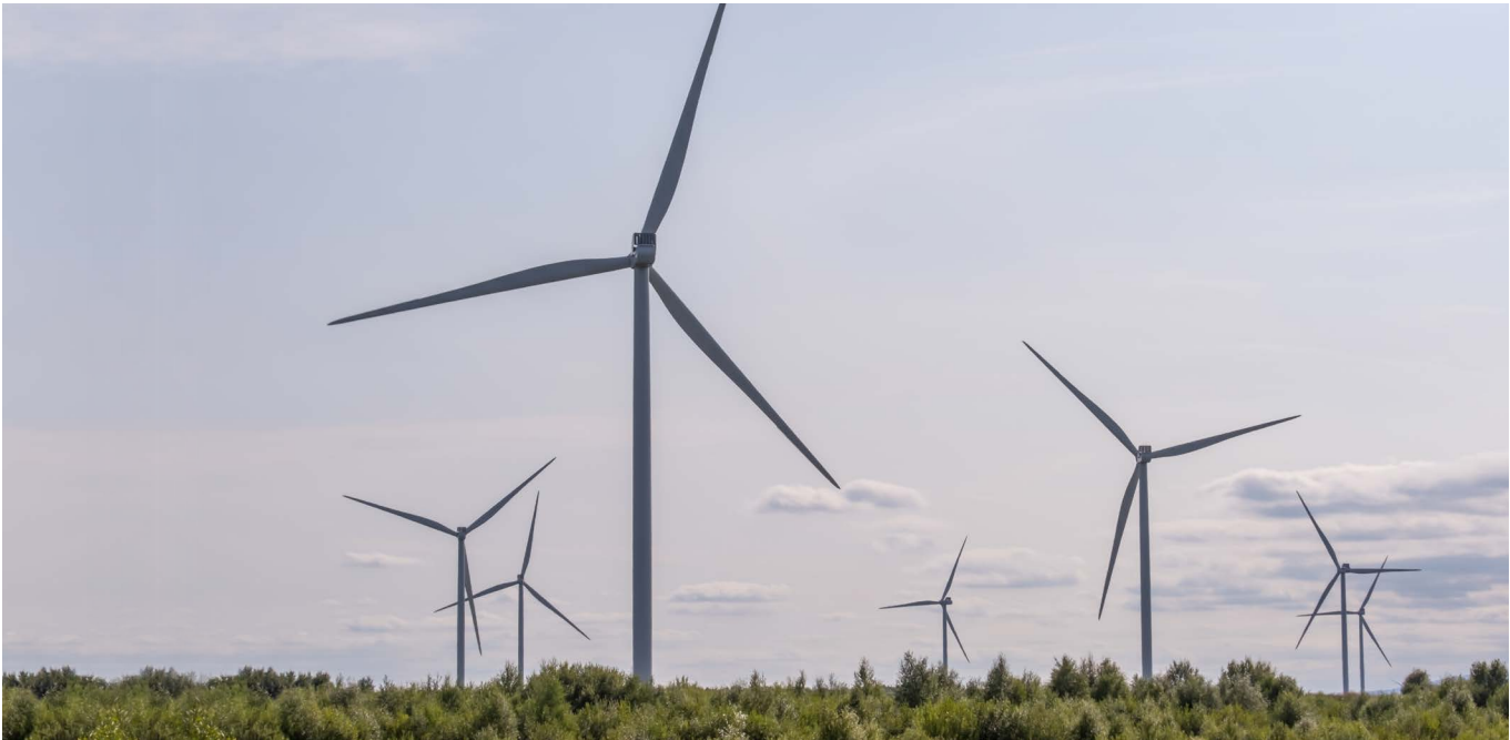
Figure 2 Cloncreen Wind Farm, County Offaly
