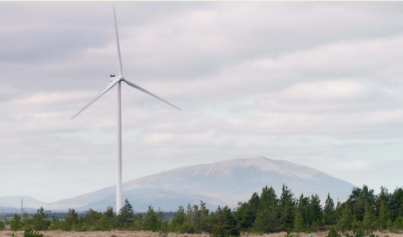
Figure 30 Oweninny Wind Farm, County Mayo (Joint Venture partnership with ESB)
