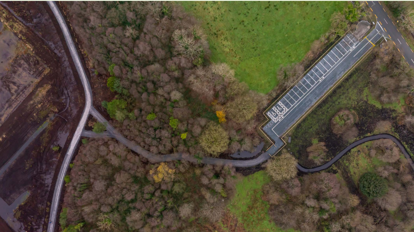
Figure 15 A woodland feature trail connects the accessible car park to the core trail at the Ballyforan Greenway in County Roscommon.
